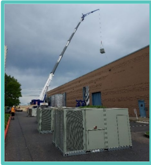
New HVAC equipment installed on the Fleet Warehouse roof
