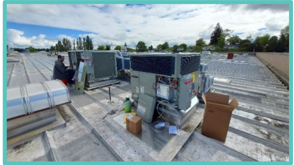
New HVAC equipment installed on the Fleet Warehouse roof
